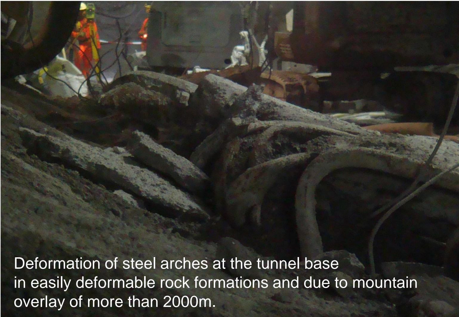
Deformation of steel arches at the tunnel base
